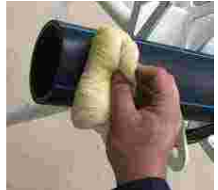
3-Clean pipe scraped area . Note: do not touch the scraped area with bare hands after scraping and cleaning.
