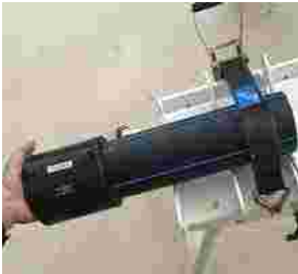
4- Insert pipe into electrofusion coupler.
